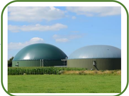
Anaerobic Digester Consider: Is this a legacy digester?
